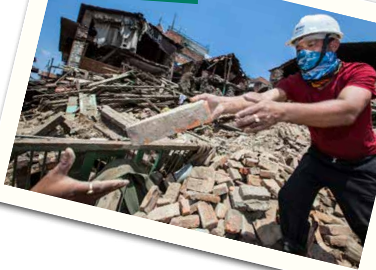
Rubble removal in Nepal
